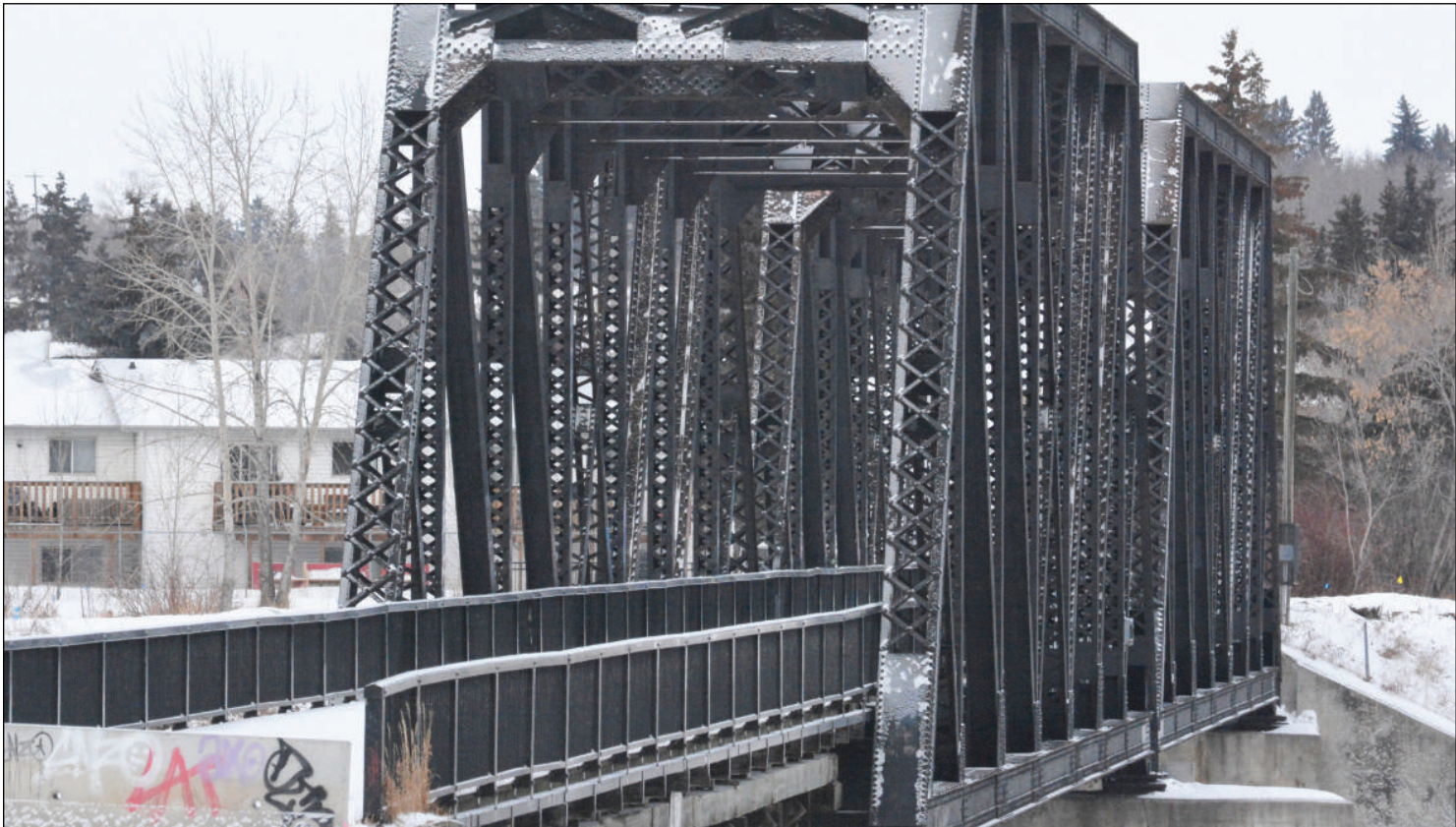
The City of Red Deer is ramping up rehabilitation of the CPR pedestrian bridge in Red Deer this week. (Advocate file photo)
